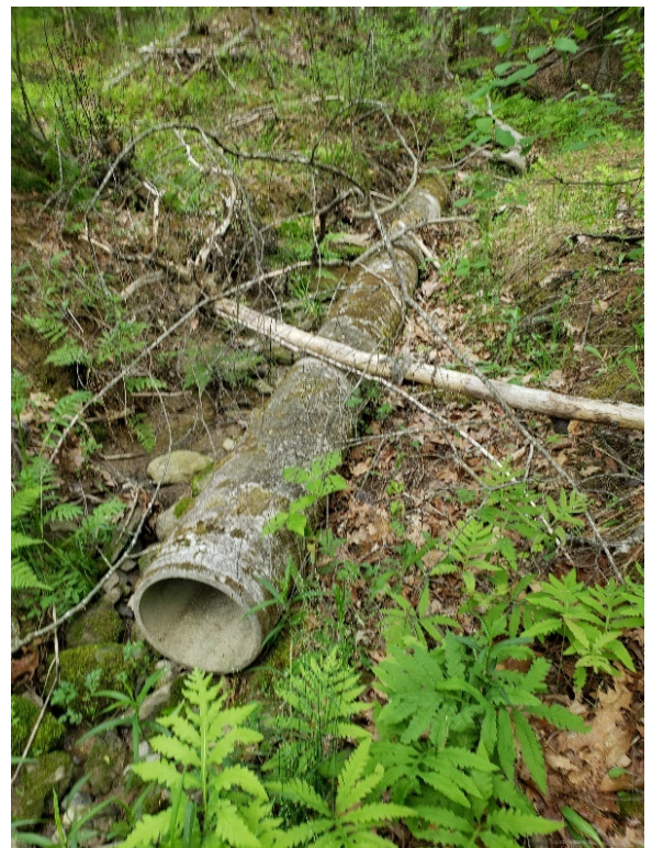
Photo 10: Concrete culvert observed in sitting in the channel of Stream 6.
